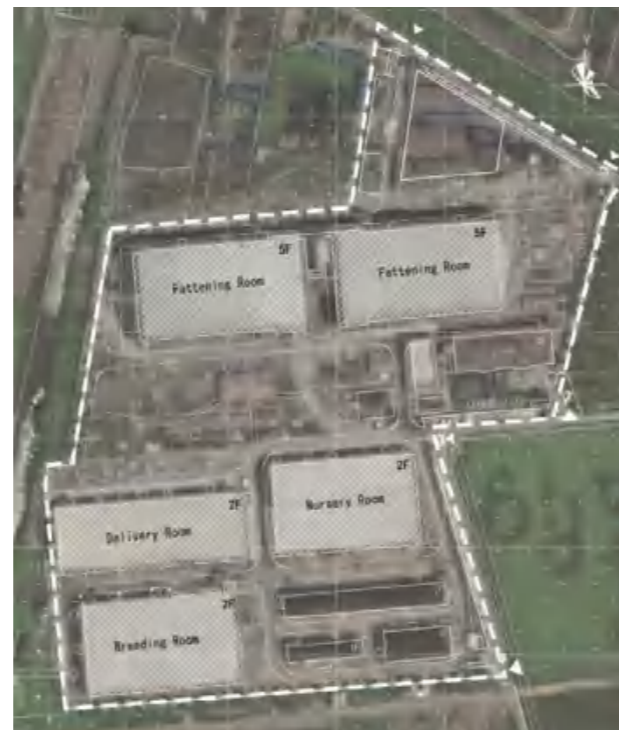
Figure 5-1-3-6 PV panel installed roof of Huasheng Ranch
