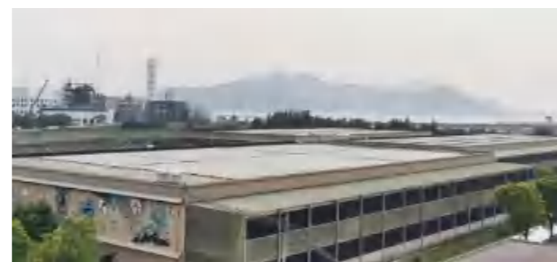
Figure 5-1-3-5 PV panel installed roof
