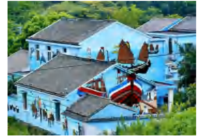
Figure 4-3-7 Two-storey brick structure
