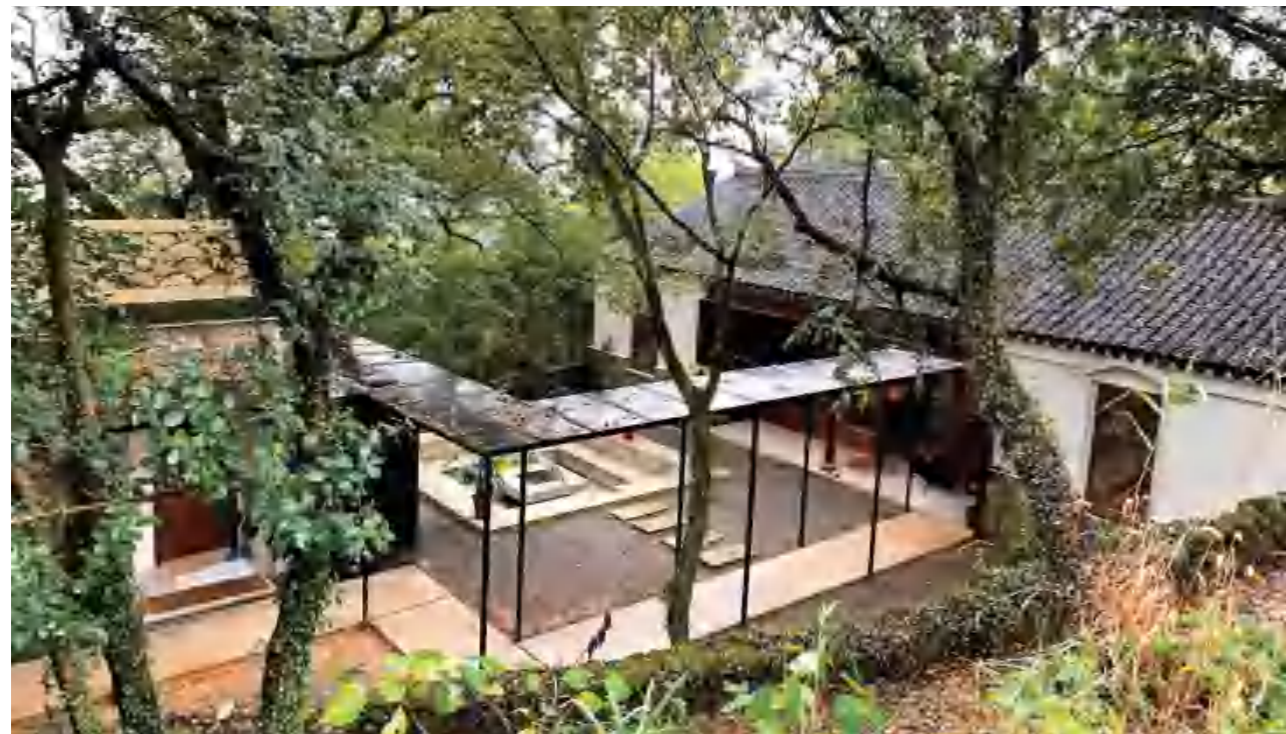
Figure 5-3-2-1 Hostels converted from vacant houses
