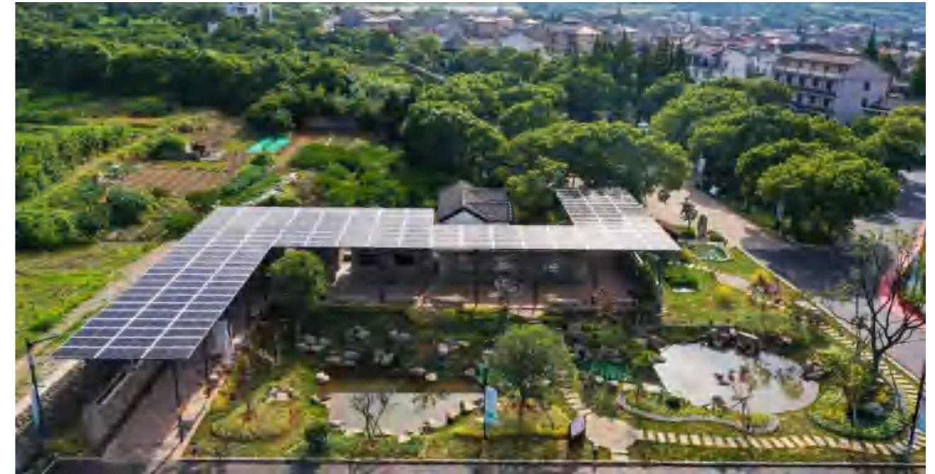
Figure 5-1-2-4 PV installed roof
