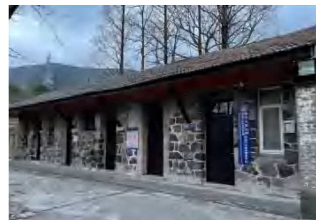
Figure 5-3-2-6 Front of the barracks and its building material
