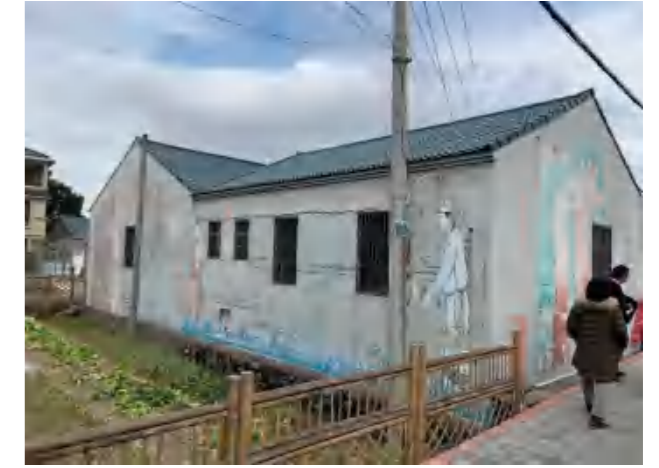
Figure 4-3-6 One-storey brick structure
